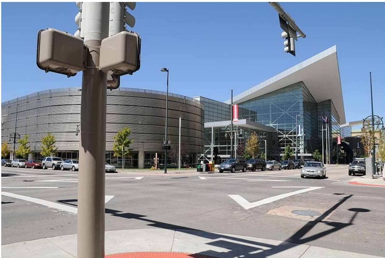
Kolorado kongresni centar , Denver, USA, arh. Curtis Fentress and architects, 1977.g.
