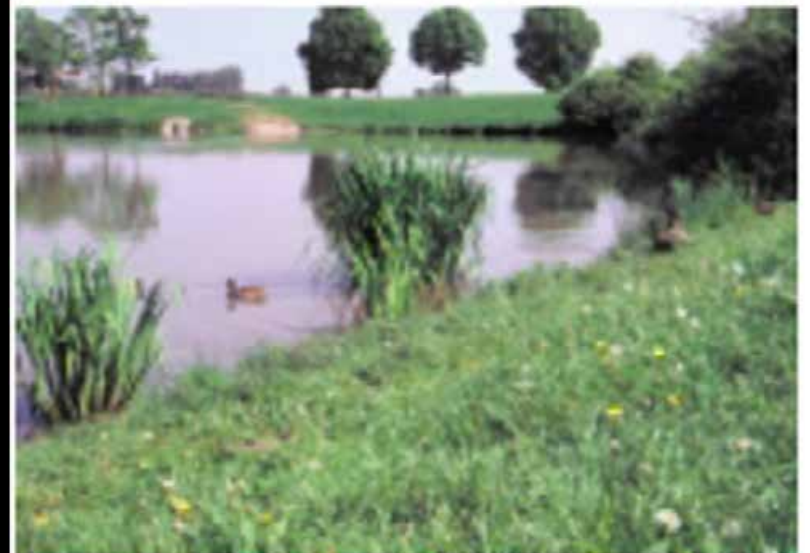
Rainwater reservoir Anecamp
