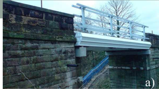
a) Prosta greda, Anegasakigava most, Japan
