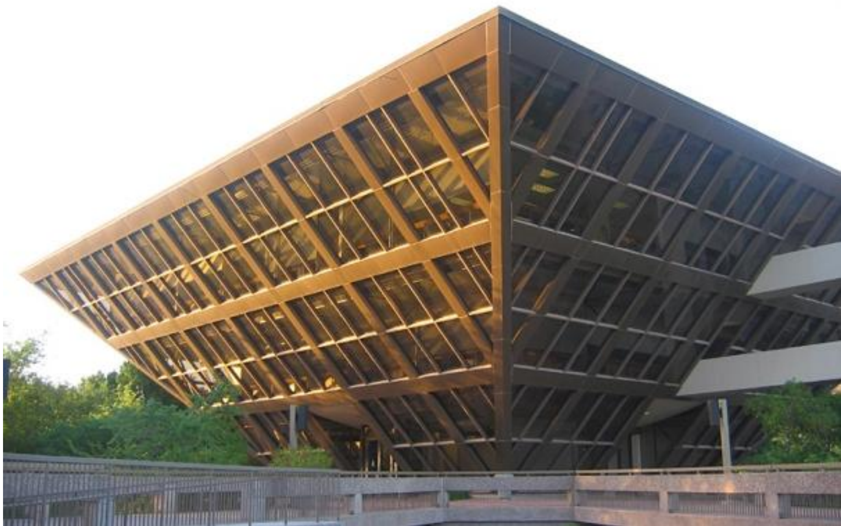
Tempe Municipal Building , Tempe, Arizona, SAD, arh. Majkl i Kemper Gudvin, 1970.g
