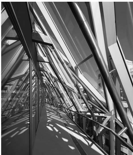
Slika 1 – Dvostruka fasada na objektu Basque Health Department Headquarters u Bilbao
