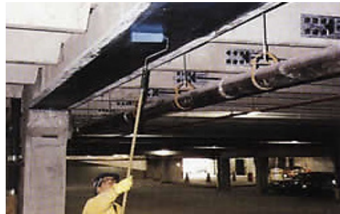
Figure 14. The application of flexural strengthening, [21]
