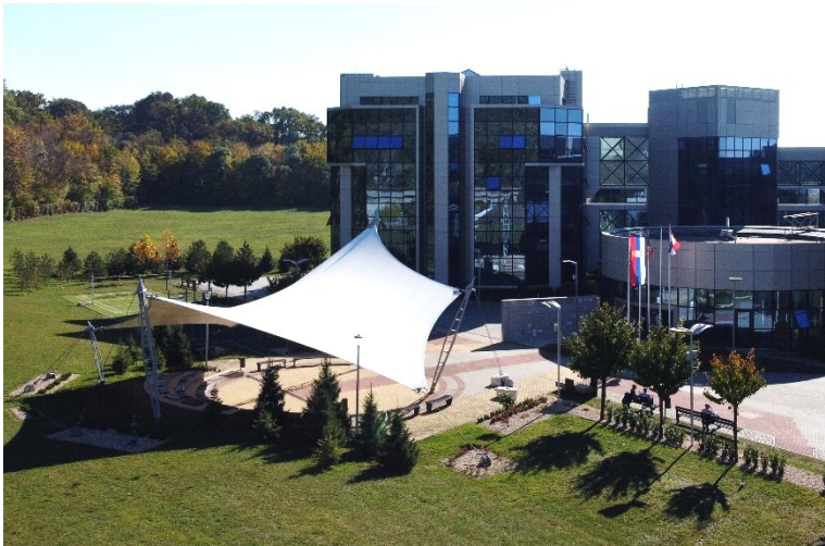
Figure 1. Tensioned membrane at the Science and Technology Park Belgrade, by Artech (courtesy of www.artech.rs )
