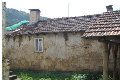
Figure 6. Northeast façade of the house, source: authors
