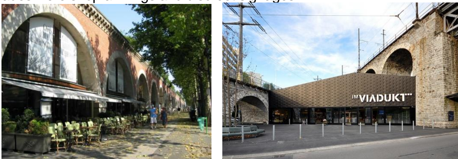
Figure 1. Two types of interventions – filling the arches (left, Viaduc des Arts) vs. adjacent construction (right, IM Viadukt), Wikipedia Commons
