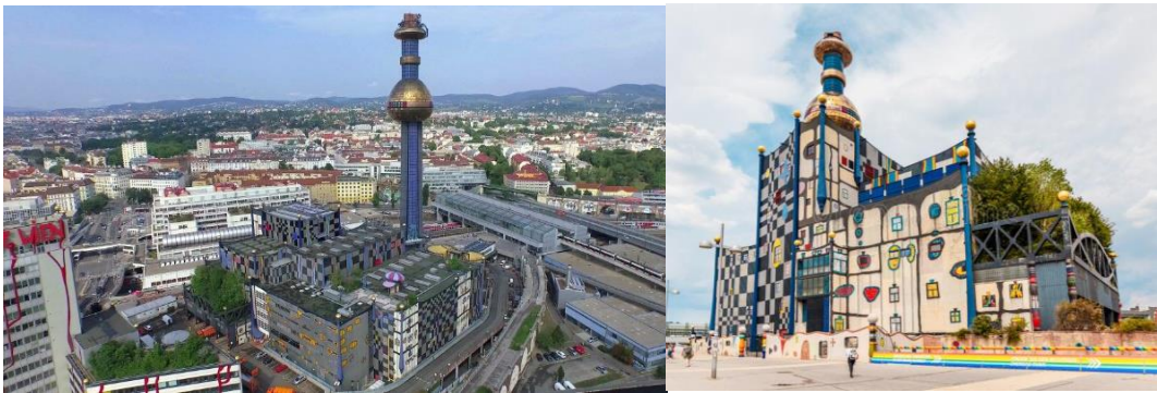
Figure 1 and 2. Spittelau incinerator, Vienna, Austria
