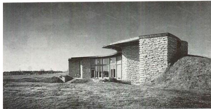
HERBERT JACOBS HOUSE II IN COUNTRYSIDE NEAR MADISON, WIS. TWO-STORY SOLAR HEMICYCLE BANKED AGAINST WIND.
