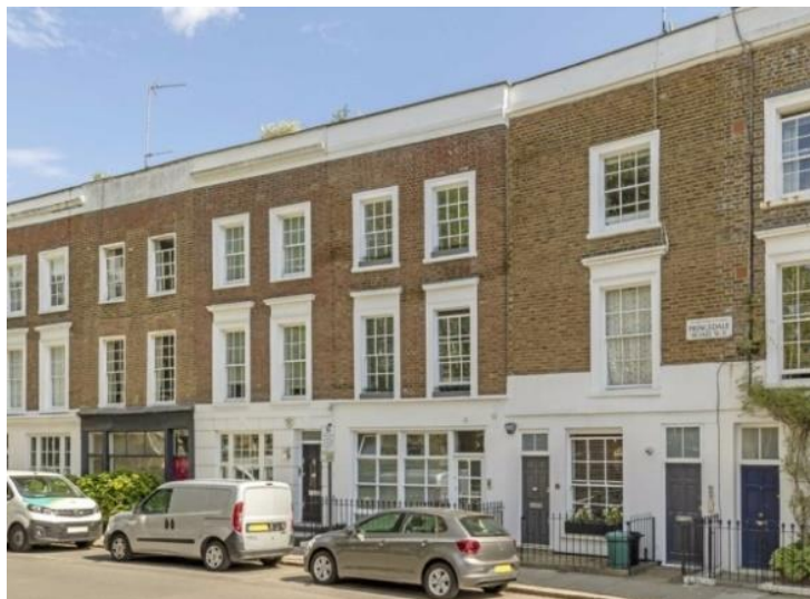
Figure 3: „Holland Park Home“, after conversion [15]
