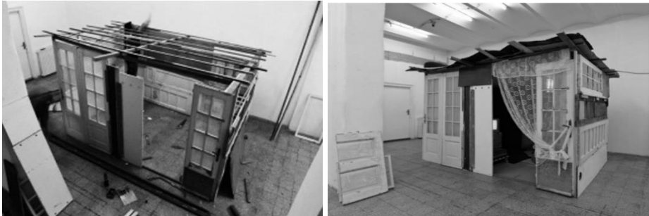
Figure 2. Demonstration of a dilapidated house.
