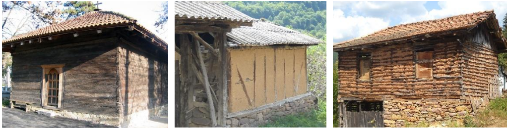
Figure 1. Left-“daščara” church in S. Palanka, in the middle-“bondručara” in village Senokos, right – “čatmara” in village Senokos (Sources: https://sn.rs/nrbso ; authors)
