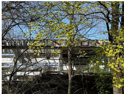
Figure 8. The Luminous Sign Covered and the Stairs Ruined ,personal photo, April 2022
