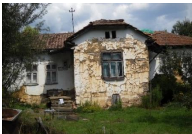
Figure 5. Southwest façade of the house, source: authors
