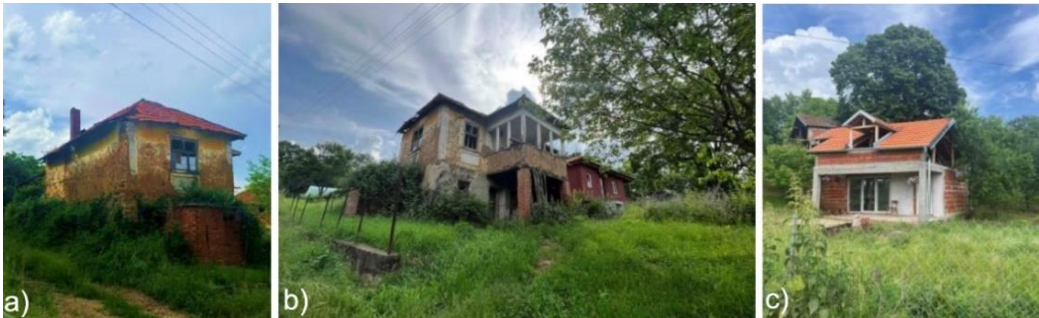
Figure 4. a) Old and abandoned village house, b) an example of a new house next to the old one, c) new house under construction, source: personal archive, May 2023
