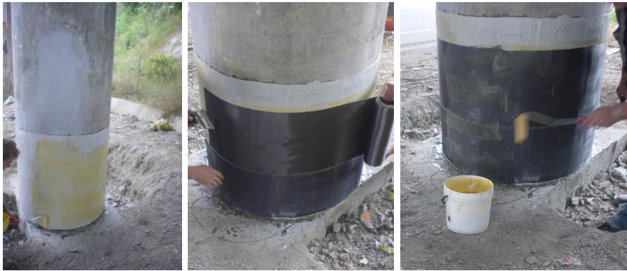
Figure 3. Confinement strengthening (Di Ludovico M.[3])
