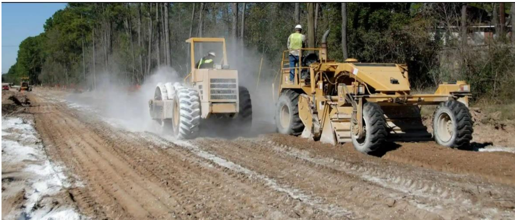
Figure 1. The chemical soil stabilization technique
