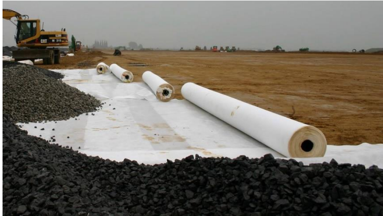
Figure 1. Geotextile in road construction, source: https://mc-plus.hr/novosti/blog/gradevinski-materijal-geotekstil-43/ (8.6.2023)
