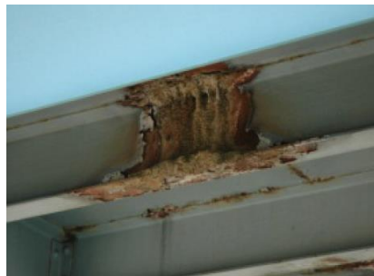
Figure 9 – Chemical damage [16]
