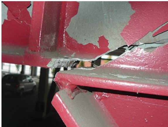
Figure 3 – Brittle fracture [11]
