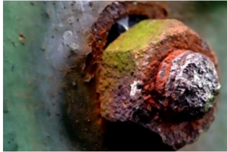
Figure 23 – Bacterial corrosion
