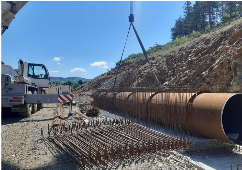
Figure 4. Installation of steel pipe
