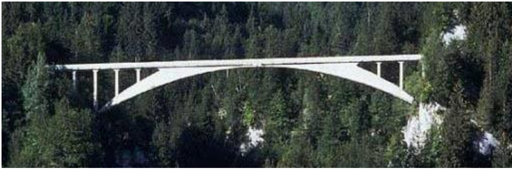
Figure 1. Salginatobel Bridge , Switzerland (Maillart) 1929/30, after [1]
