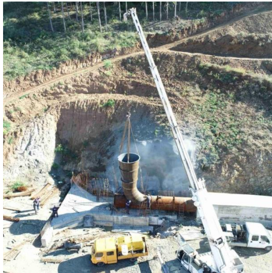
Figure 6. Installation of a cone for entrance construction
