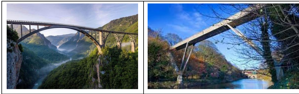
Figure 12. Djurdjevica Tara Bridge, Montenegro, M. Trojanovic, 1939.
