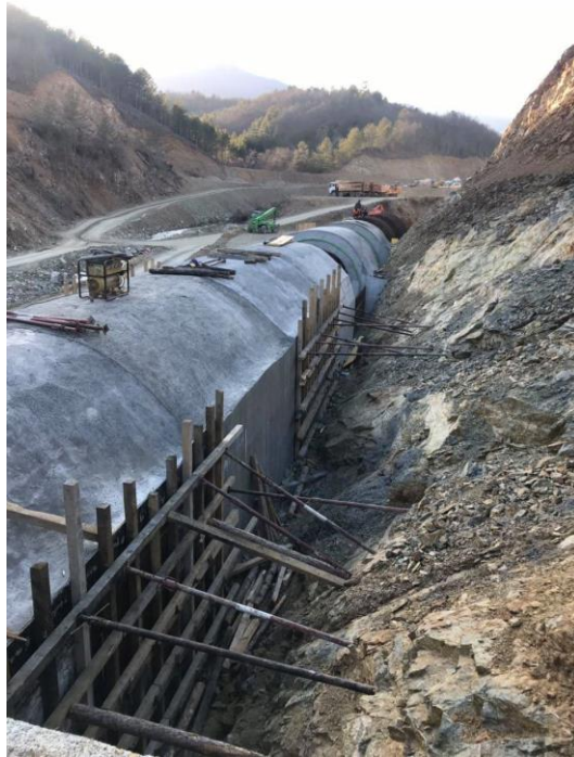
Figure 12. The diversion tunnel in construction
