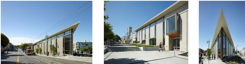
Figure 2. North Beach Branch Library Building, San Francisco, LMS Architects www.archdaily.com
