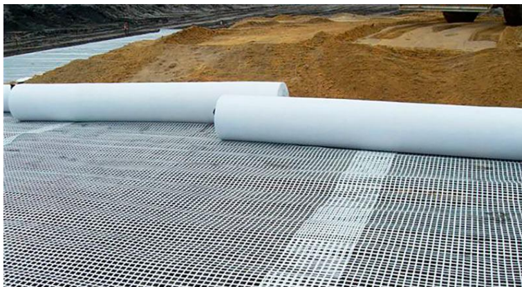
Figure 2. Geosynthetics - “geonet” in road construction, source: https://en.milford.dk/products/geonet (8.6.2023)
