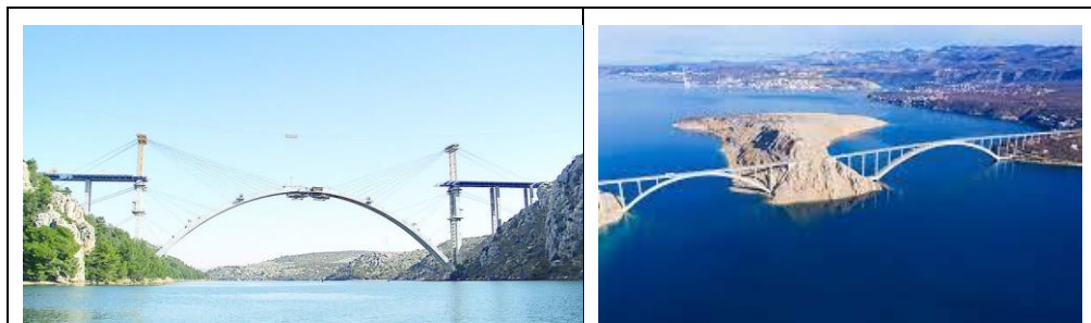
Figure 14. Bridge Krk-St. Marc-mainland, Croatia, I. Stojadinovic, 1980.
