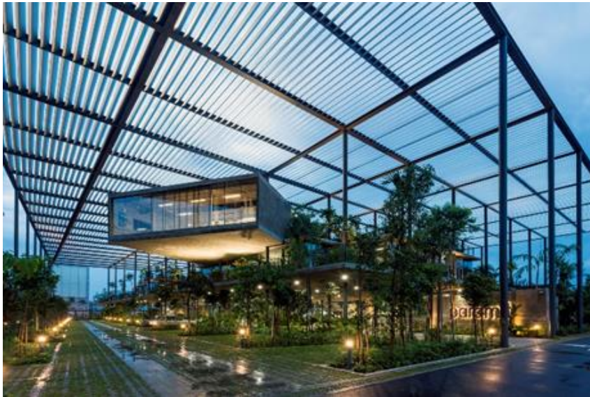
Figure 1. Factory in the Forest, https://www.archdaily.com/947771/factory-in-the-forest-design-unit?ad_medium=gallery
