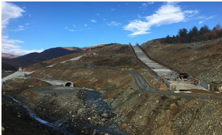
Figure 13. Diversion tunnel exit
