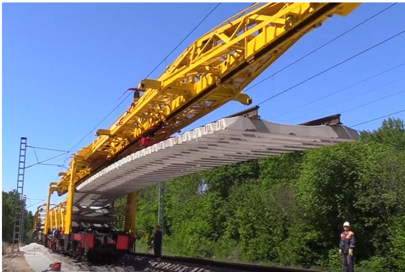
Figure 2. An example of ready-made field's method for sleepers setting down [13]
