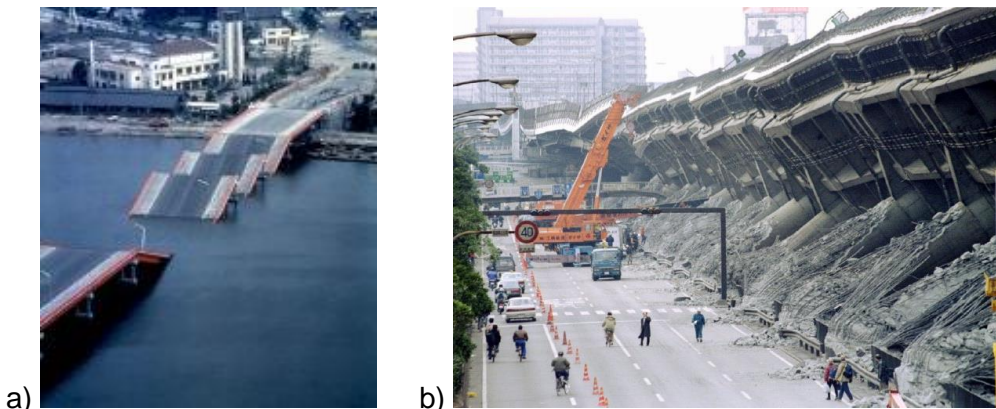
Figure 1. a) Collapse of the Showa Bridge during 1964 Niigata earthquake, source NISEE b) Collapse of piers in Hanshin Express Highway during 1995 Kobe earthquake, source Reuters
