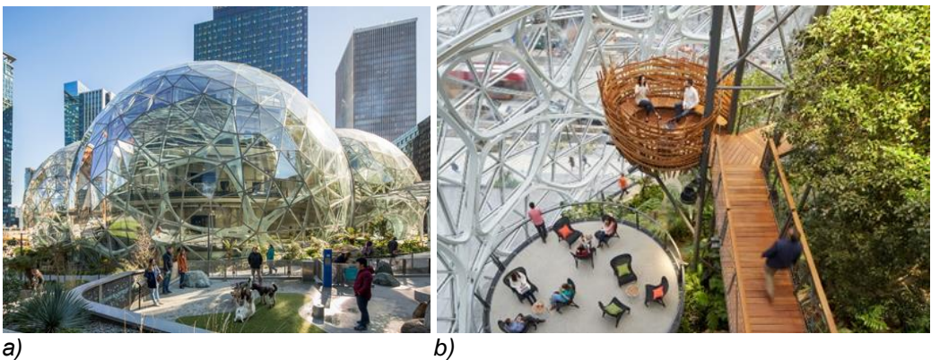
Figure 8. Amazon - the three glass spheres: a) view from outside, b) view from inside with seating areas, https://www.archdaily.com/920029/amazon-spheres-nbbj?ad_medium=gallery
