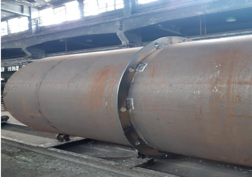
Figure 3. Welding of steel rings in a factory
