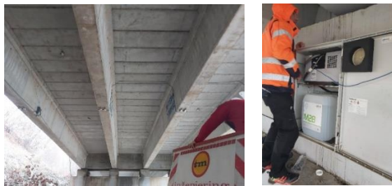
Figure 2. Installation of the SiWIM system in Serbia
